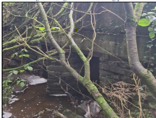
Plate 4-3 Culvert Crossing CC3
