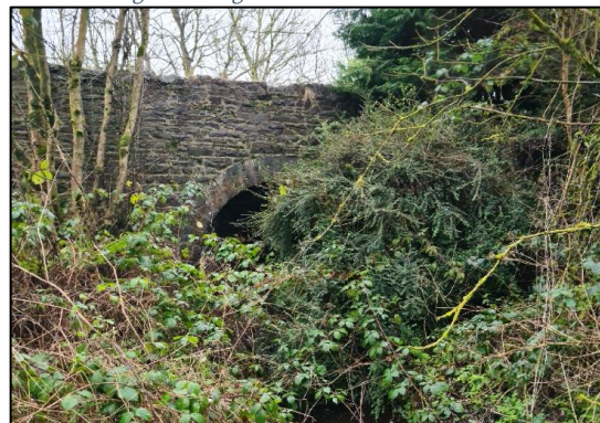
Plate 4-4 Bridge Crossing BC5, with roosting potential.
