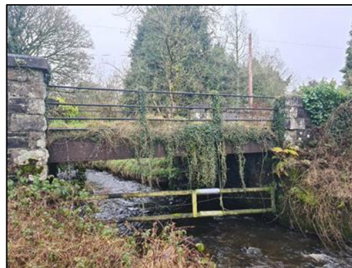
Plate 4-2 Bridge Crossing BC6
