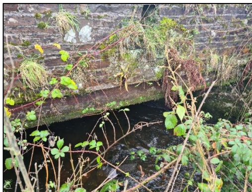
Plate 4-1 Bridge Crossing BC7 with roosting potential.
