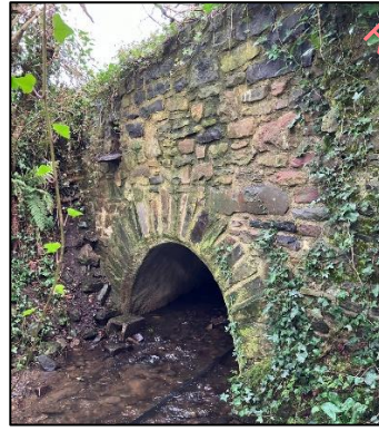
Plate 4-6. Bridge Crossing BC3
